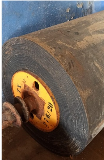
FOTO – L2-2: CORREIA TRANSPORTADORA 48’’ – 3 LONAS – COBERTURA 3/16’’ X 1/16’
